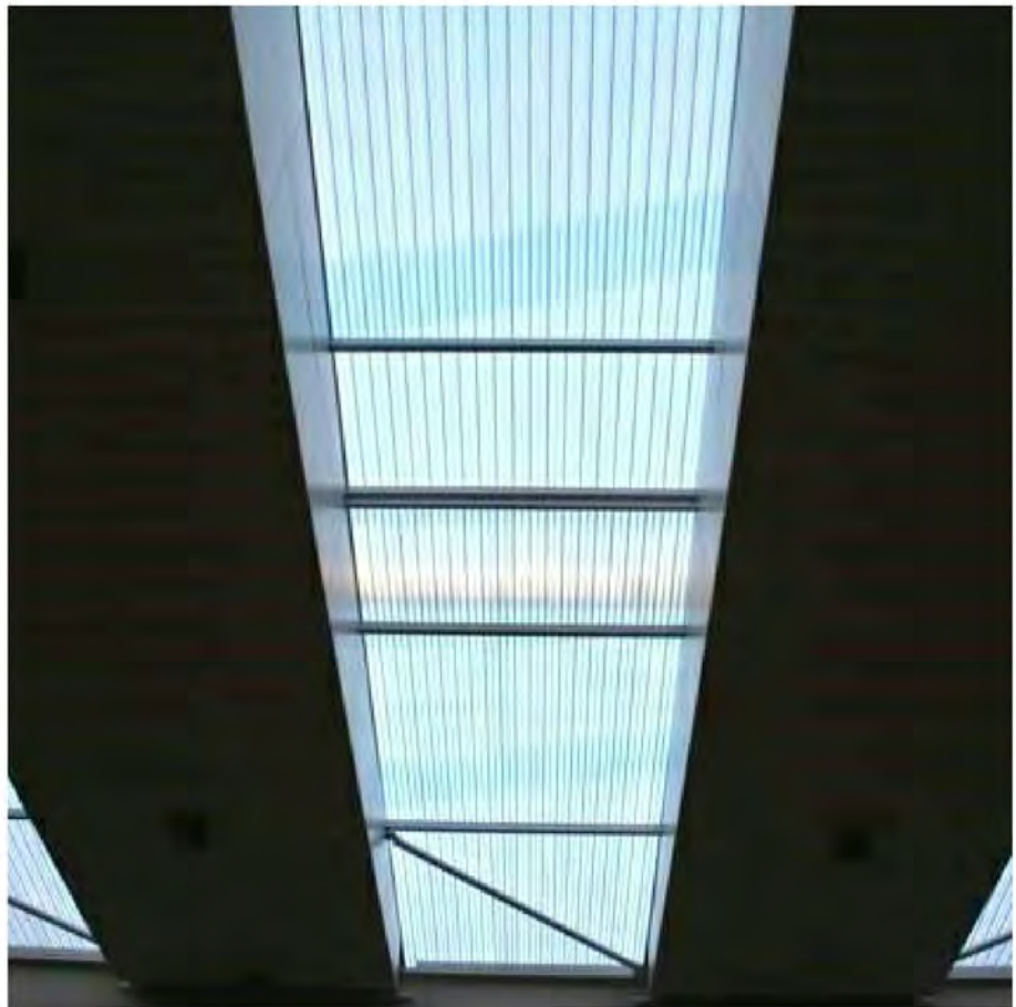
5 POLYCARBONATE ROOF SHEETING - EVERBRITE OR SIMILIAR
